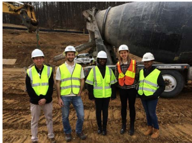
Tom Miner, P.E. and WBCM's students at the site of the City of Baltimore's new Loch Raven Dam Environmental Operations Facility
